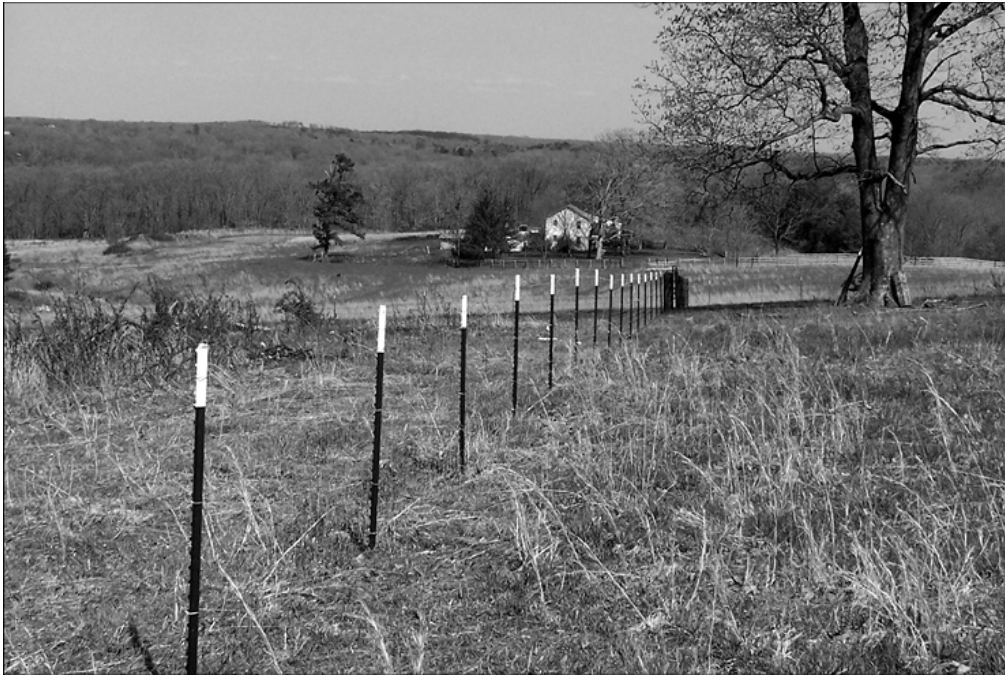
Steel T-posts like this are easy to drive and long-lasting.
